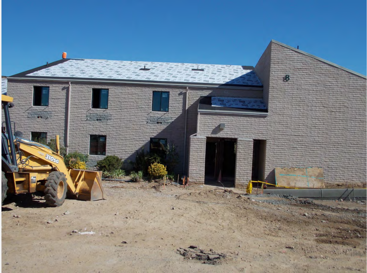
Installation of New Roof
