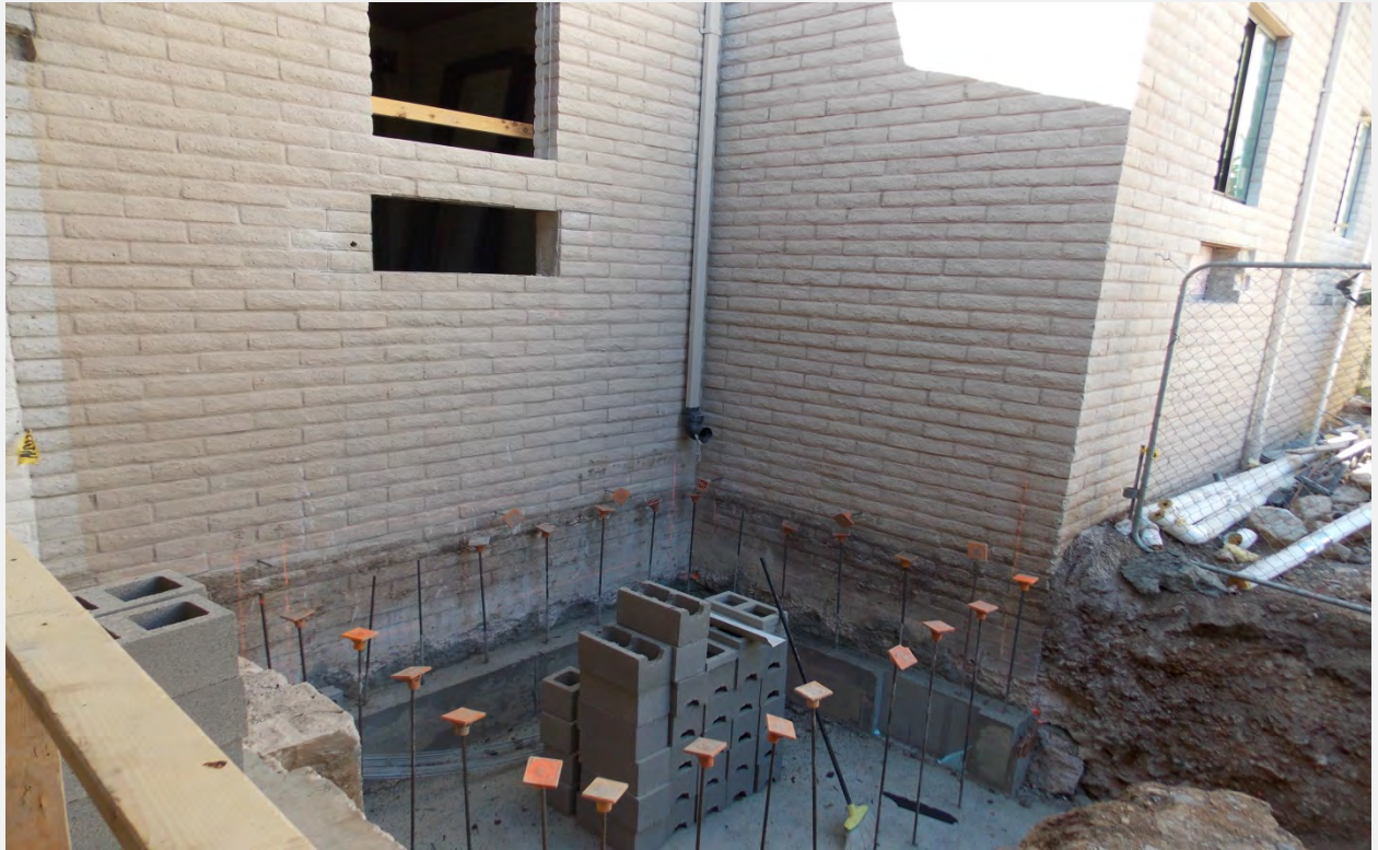
Constructing of Elevator Shaft
