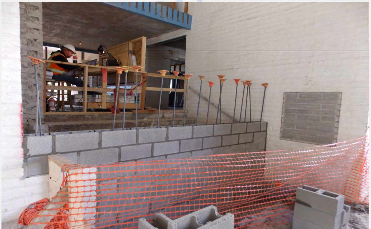
Masonry Work for New Reception Area
