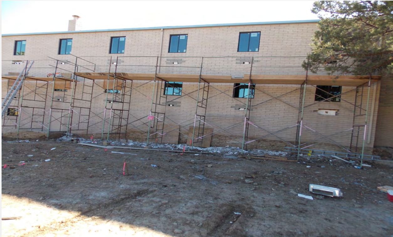
Masonry Work and Installation of New Windows
